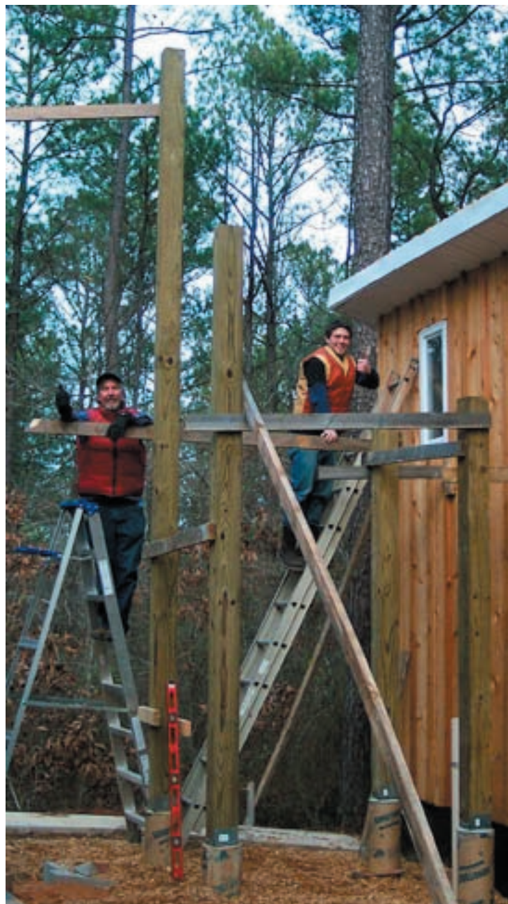
CWU-103 instructor Mark Tew (left) and his grandson, Lee Lewis, work on an elevated tank stand at the new “Mississippi” building at Camp Hopewell.
