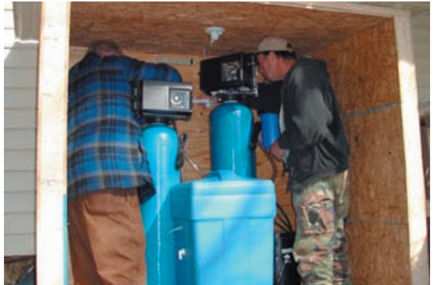
LWW volunteer Harold Iley (left) of Corbin, Ky., and Buffalo Creek homeowner Donald Shelley squeeze into a well shed to install a water treatment system. The tall tank on the right is a greensand filter, the one on the left a water softener.
